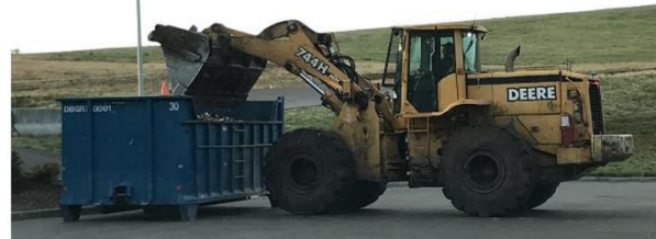
Reloaded into 30 yard box
